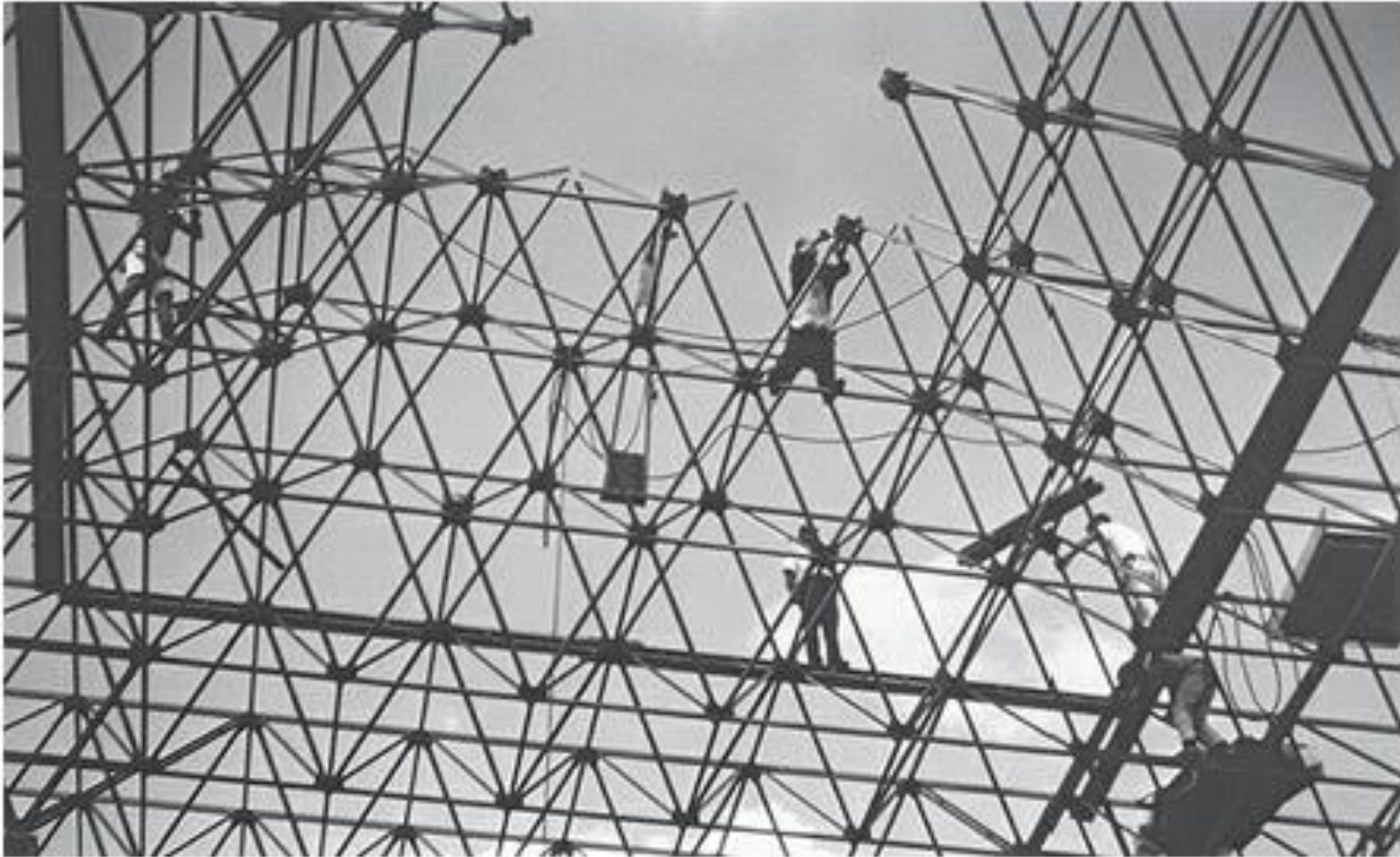
FIGURE 11.82 Assembling a space truss.
