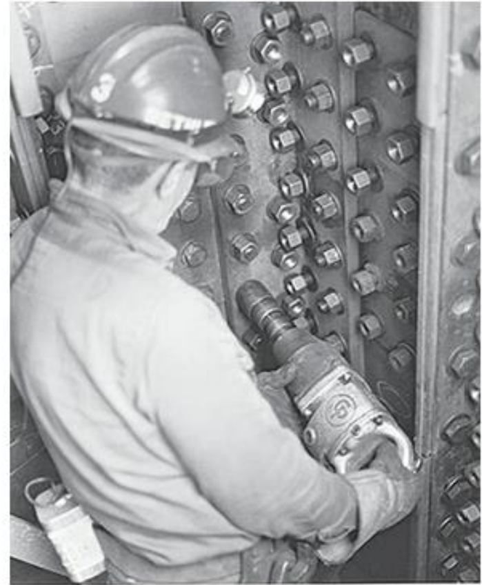
FIGURE 11.16 An ironworker tightens high-strength bolts with a pneumatic impact wrench.
