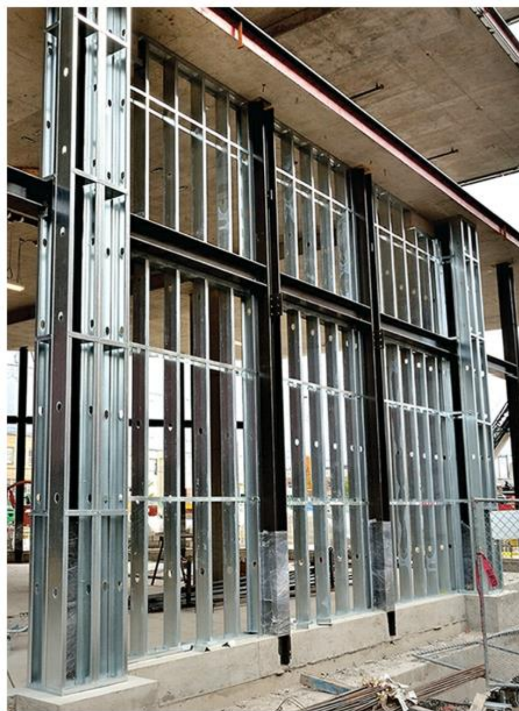
FIGURE 12.17 Light gauge steel stud infill between concrete and structural steel will support the exterior cladding. Note the horizontal rows of steel strap bracing.
